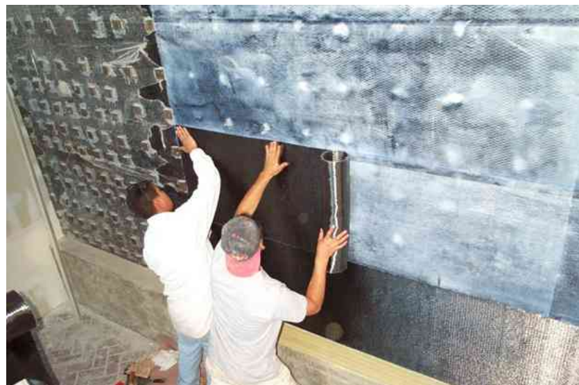
Figure 57: Strengthening of a 'shear wall' (reinforcement wall that is widely used in earthquake-sensitive structures) with carbon-composite [5]
