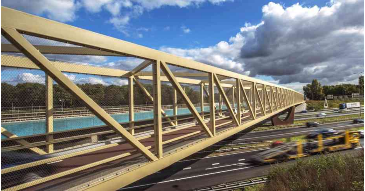
Figuur 71: Bicycle/traffic bridge crossing the Dutch highway A27; steel structure with composite deck (source: Fibercore Europe). Standards and guidelines are instrumental in ensuring optimal and safe realisation of such structures in busy traffic nodes. The challenge is to make them applicable to hybrid structures incorporating innovative materials and connections.
