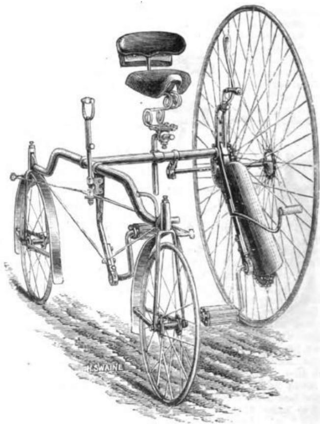
FIG. 36.—THE NEW COVENTRY ROTARY NO. 2 ROADSTER.
